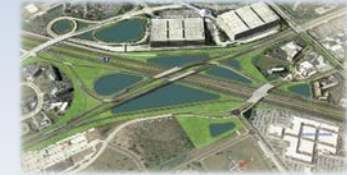
Grand National Drive Overpass / Kirkman Road Interchange
